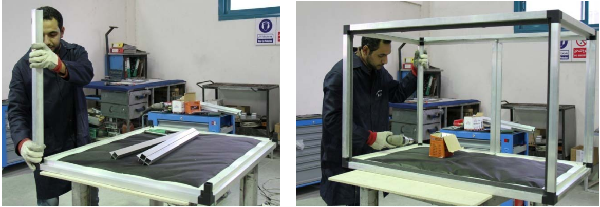
Figure 2- 2(Air handling unit casing)
