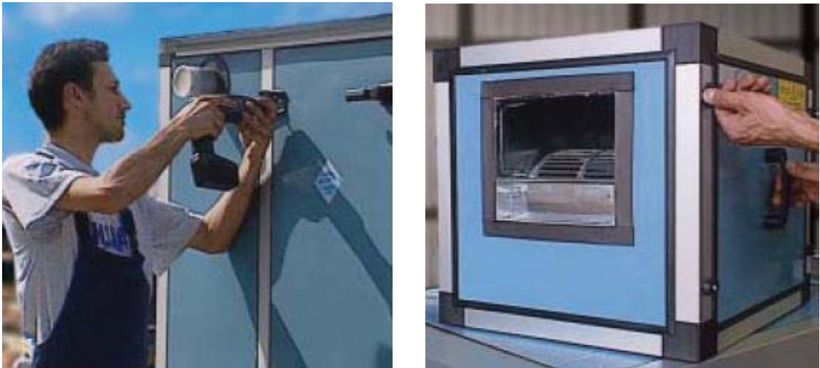
Figure 2- 4(Air handling unit inspection door)
