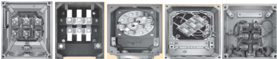
Figure 2- 45(Synchronous electric motor connections)
