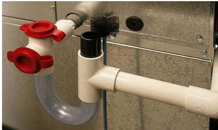
Figure 2- 23(Condensate drain trap)
