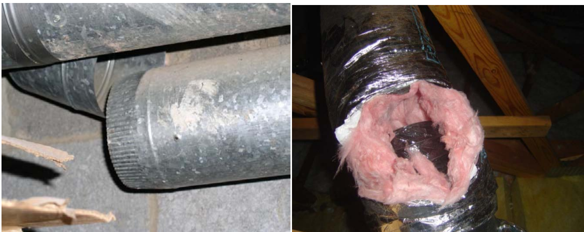
Figure 4- 5(Ducting system leak)
